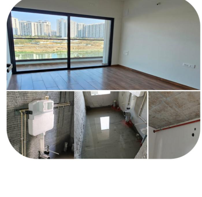
• 23rd slab gypsum plaster completed. • Plumbing work completed up to the 24th slab.
