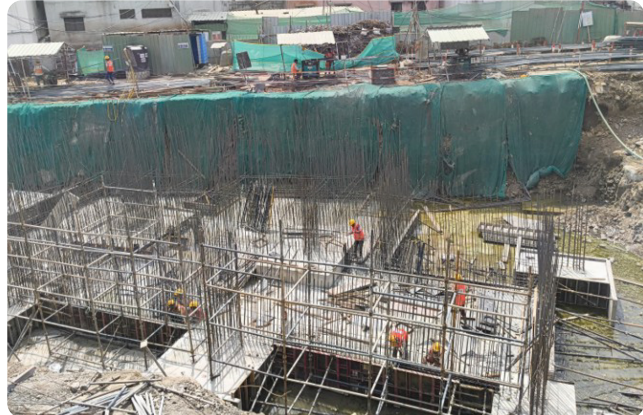
STP (Sewage Treatment Plant) Raft casting completed.
