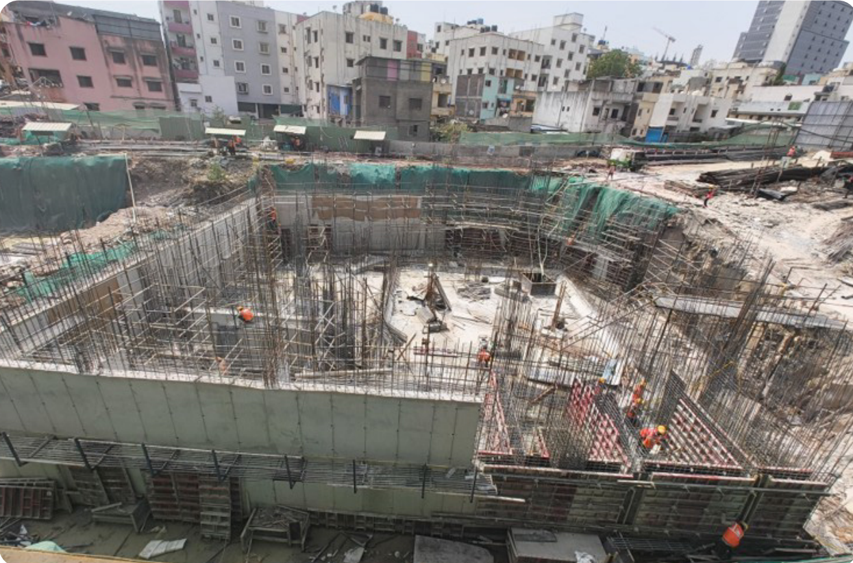
UGT (Underground Tank) RCC work in progress.
