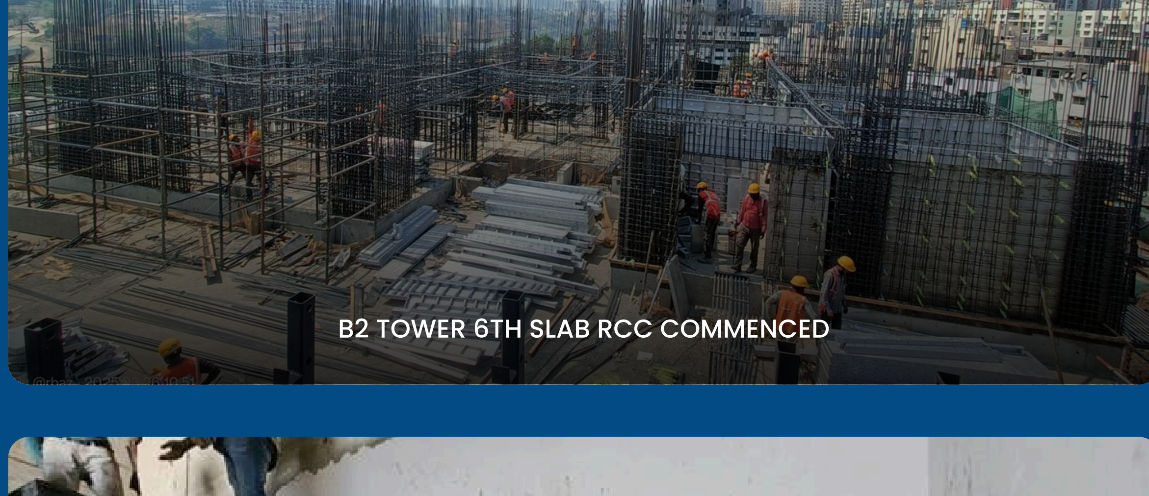
B2 TOWER 6TH SLAB RCC COMMENCED
