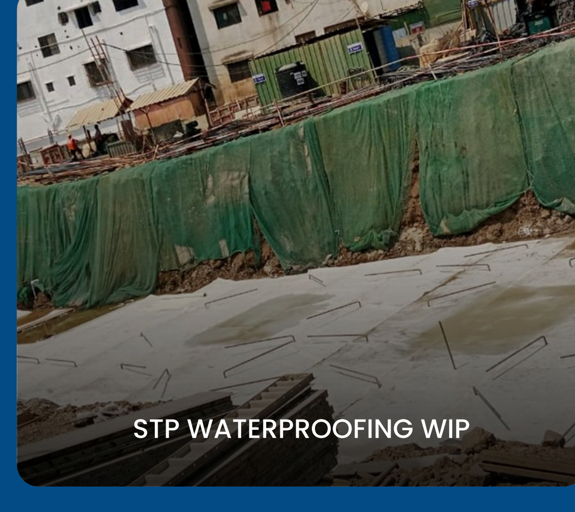
STP WATERPROOFING WIP
