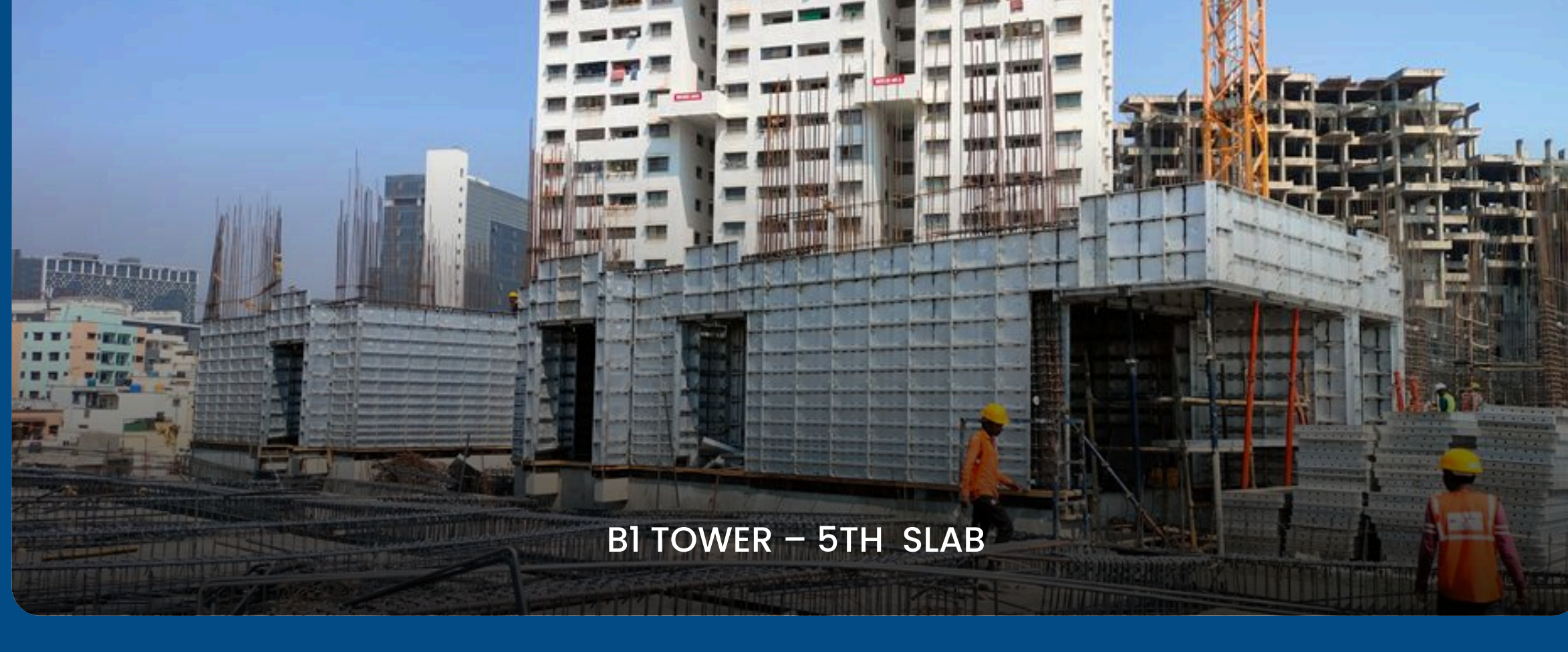
ALUFORM SHUTTERING WORK HAS COMMENCED
