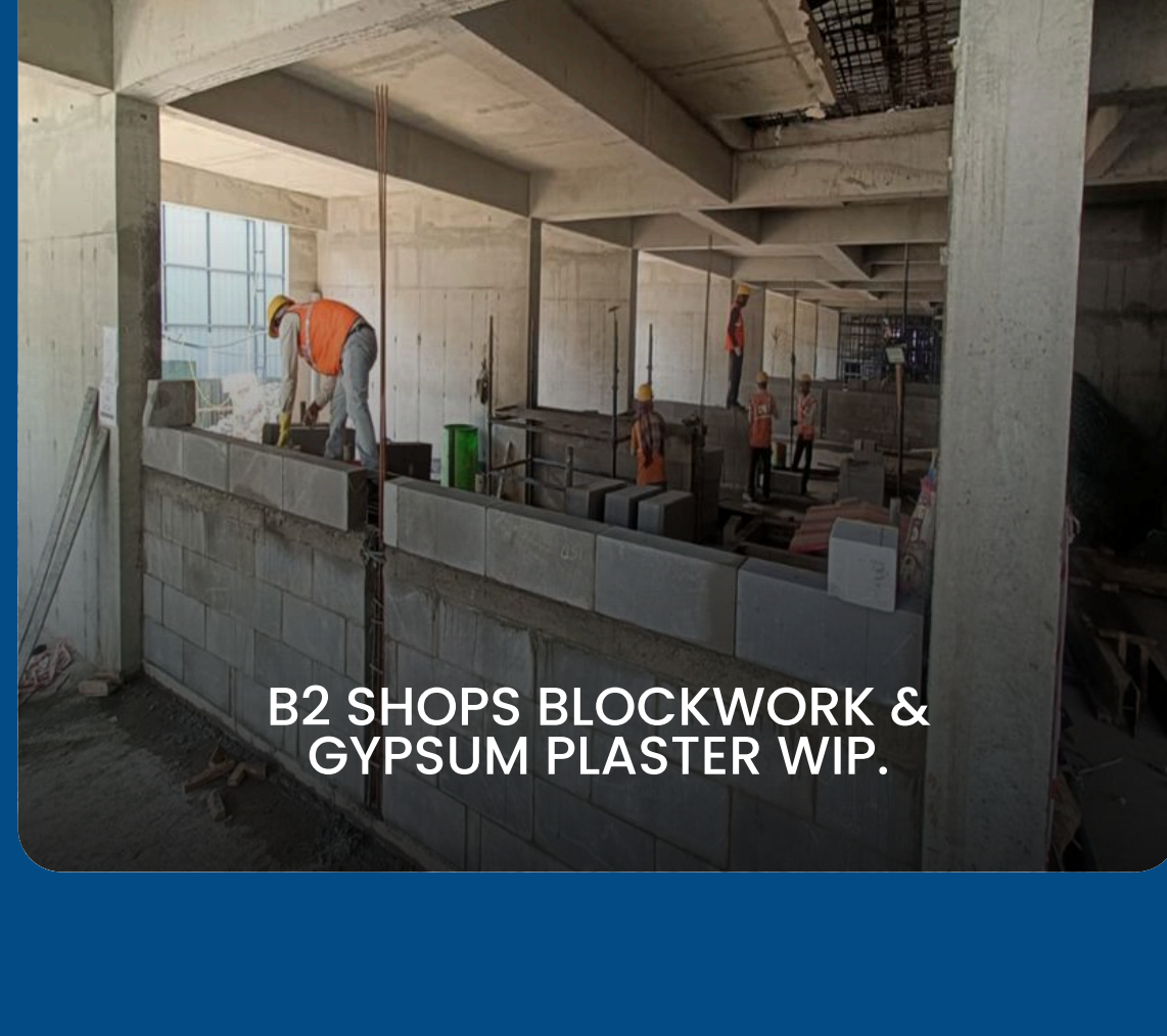
B1 SHOPS BLOCKWORK COMPLETED, GYPSUM PLASTER
